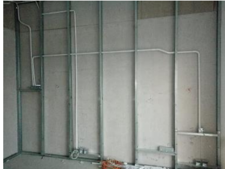
Single Layer Single side Board Work
