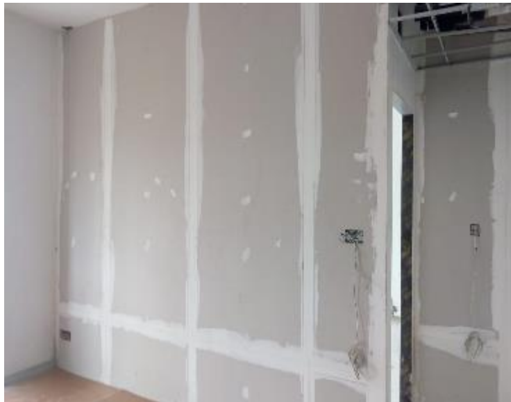
Jointing Completed Partition Work
