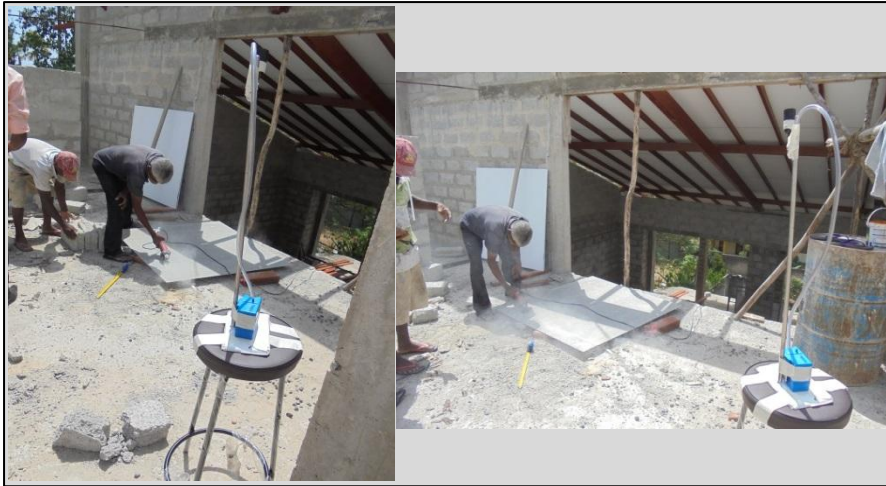
Figure 56: Air sampling of the Cutting area – 5C1
