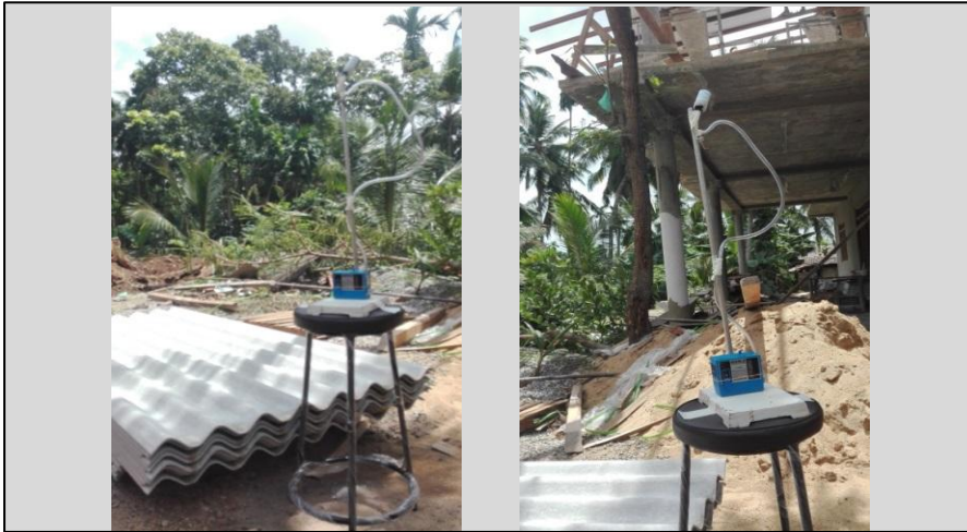
Figure 47: Air sampling of the Cutting area – 2C1
