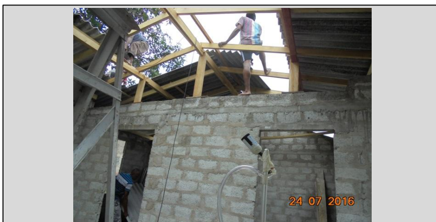
Figure 50: Air sampling of the Cutting area – 3C1
