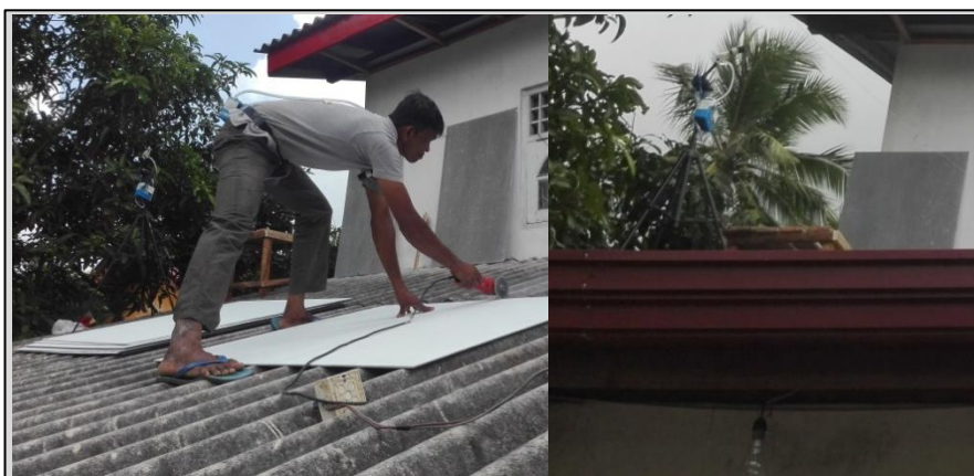
Figure 53: Air sampling of the Cutting area – 4C1
