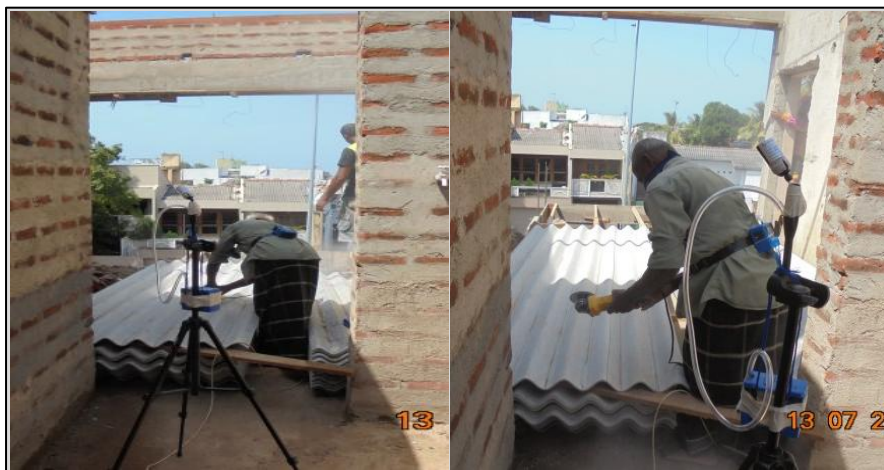
Figure 44: Air sampling of the Cutting area – 1C1
