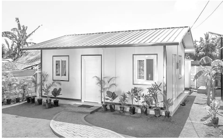
Figure 36: GI roofing sheet used house model by National housing authority The Sri Lankan national housing authority has lead a 65,000 housing programme with GI roofing sheets thinking it's a good alternative for asbestos. However, there are pros and cons of altering asbestos with GI sheets.
