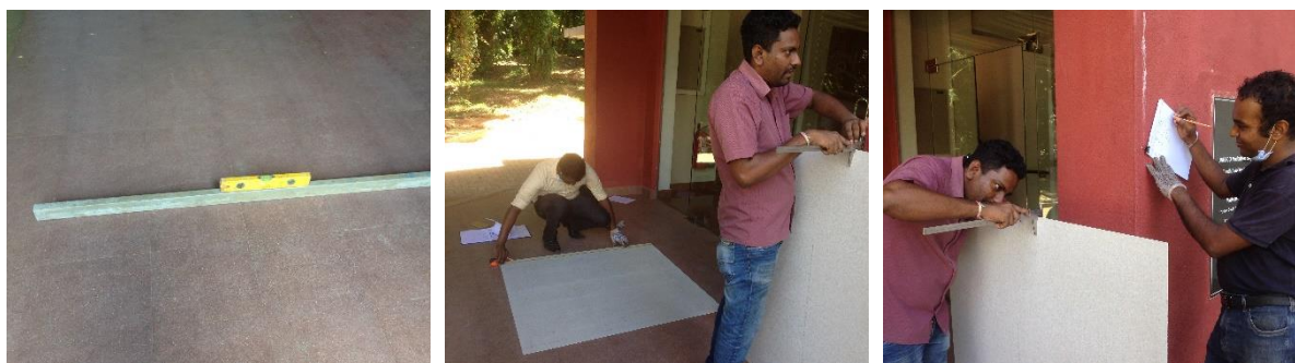
Figure 10: Preparing full sheets for taking dimensions.
